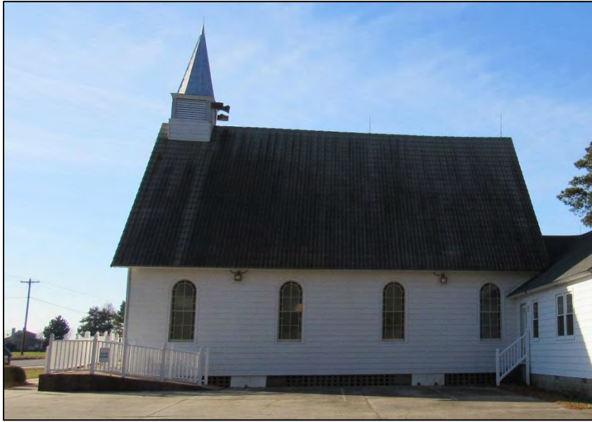
Photo 70: McBride United Methodist Church, Primary Entry Detail (Top) and East Elevation (Bottom).
