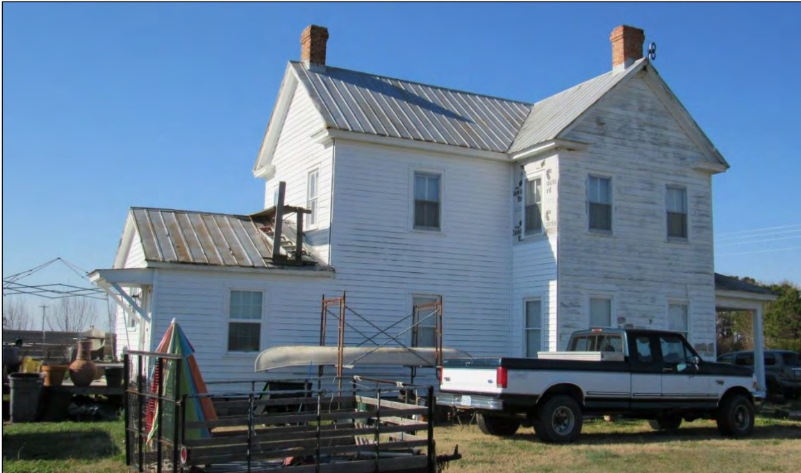
Photo 56: Northeast Elevation of the Pritchard House, Looking West.
