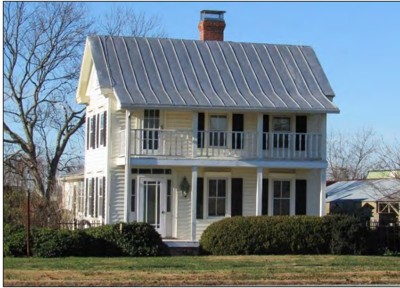
Photo 43: Southeast Oblique of Simmons-Morris House (CK0331).
