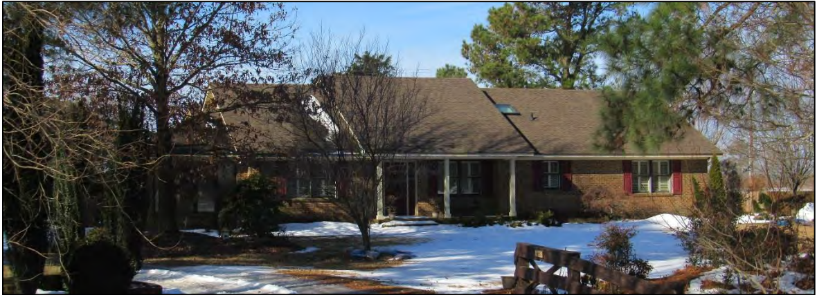
Photo 40: Circa-1985 Secondary Dwelling, East Elevation.
