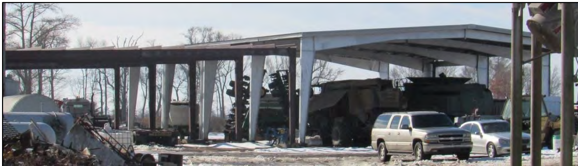
Photo 29: View of Circa-2000 (Right) and 2017 (Left) Equipment Shelters, Looking South.
