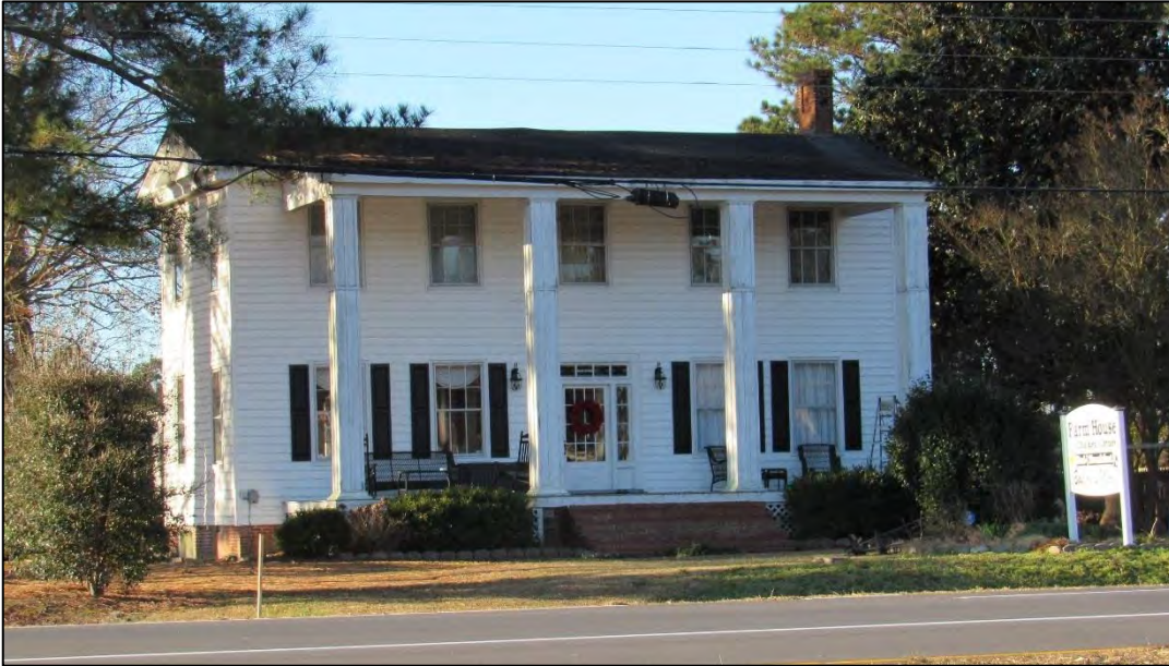
Photo 41: Primary (Northeast) Elevation of the Whitehurst-Smithson House (PK0998).
