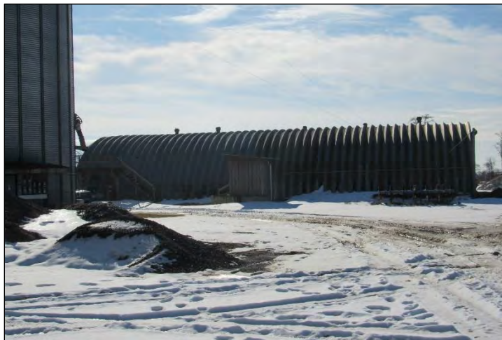
Photo 27: Quonset Hut, North Elevation.
