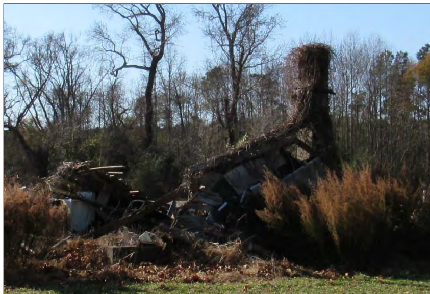
Photo 51: Frame Building Ruins, Looking Southeast.
