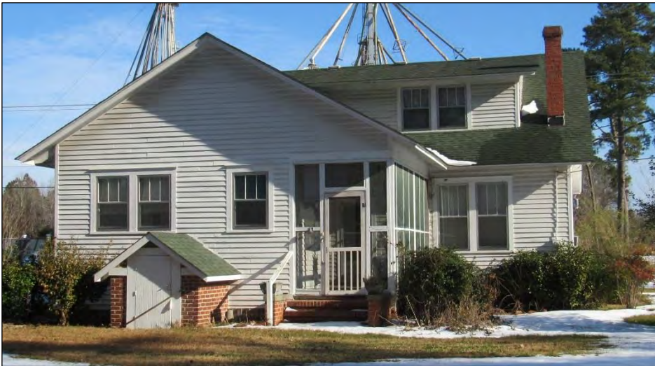
Photo 5: Southwest Elevation of the Stafford-Purden House.
