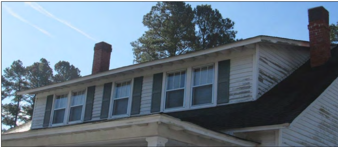
Photo 2: Detail of Dormer Along Façade, Facing South.
