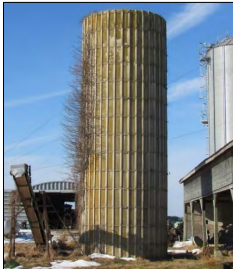
Photo 32: Circa-1950 Silo, Looking West.
