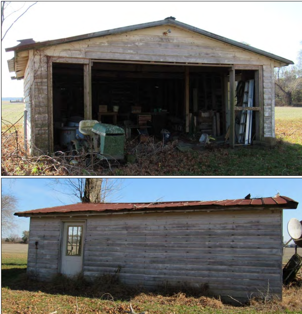
Photo 49: Garage, North Elevation (Top) and West Elevation (Bottom).
