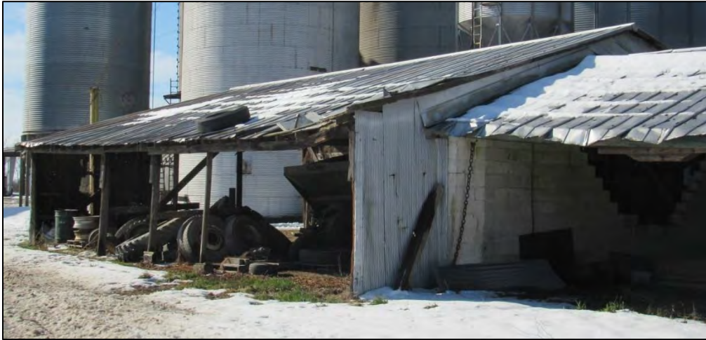
Photo 35: Circa-1965 Machine-Shed Addition, Northeast Oblique.
