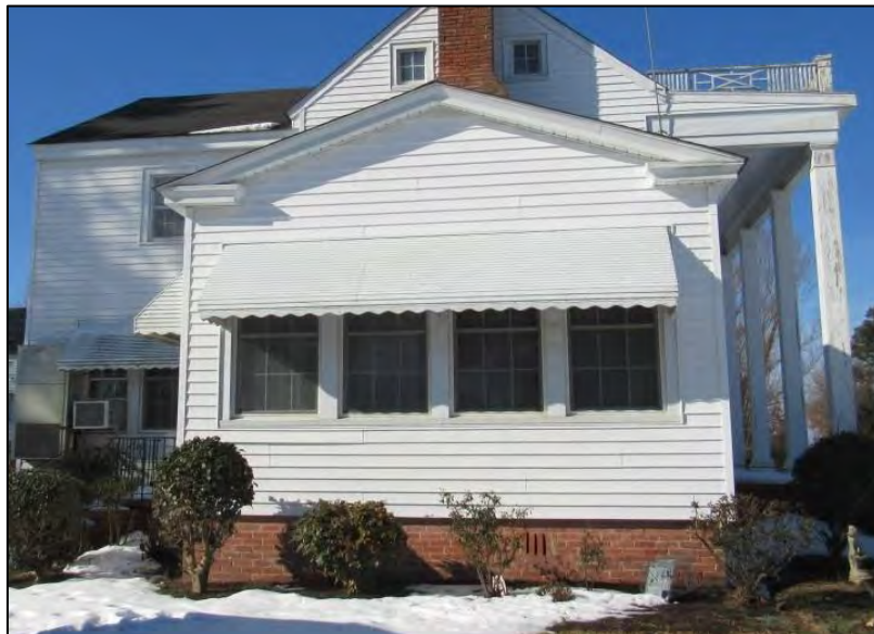
Photo 21: Enclosed Side Porch, East Elevation.
