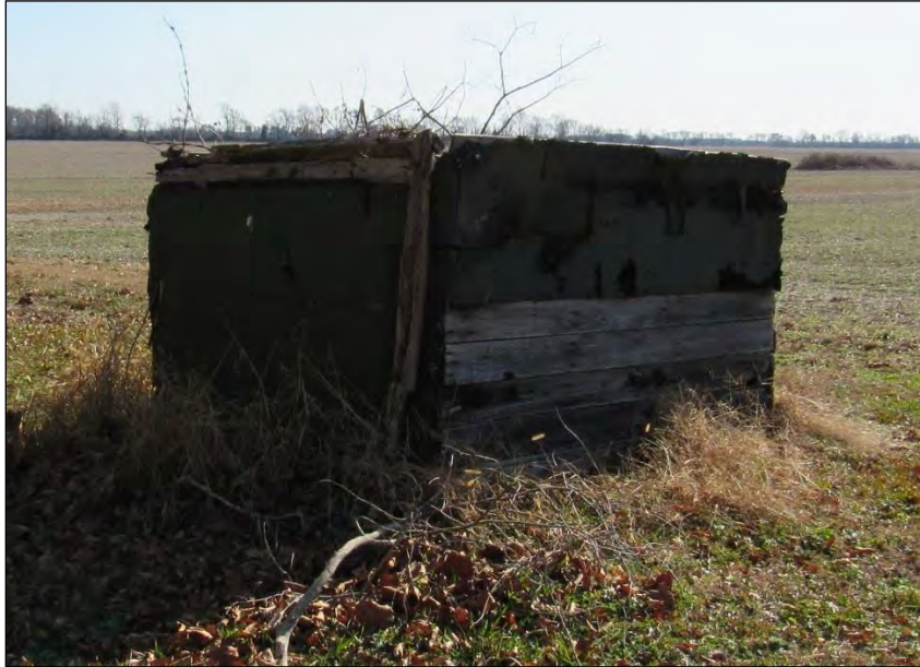
Photo 50: Well Enclosure, Northeast Oblique.
