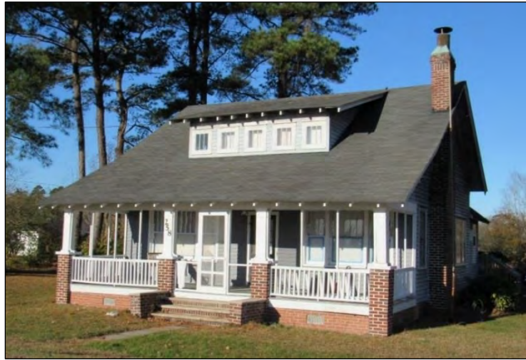
Photo 7: East Oblique of the Creekmore House (CM0074).
