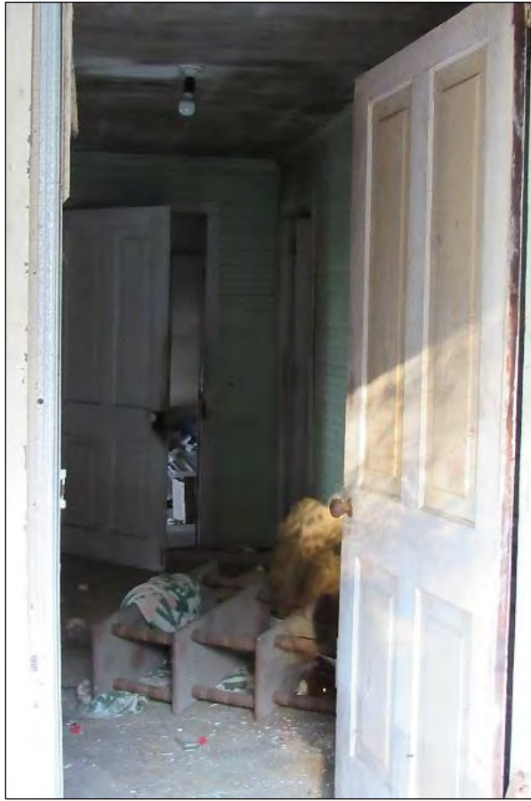
Photo 66: Primary Entrance on the East Elevation of the Griffin House.
