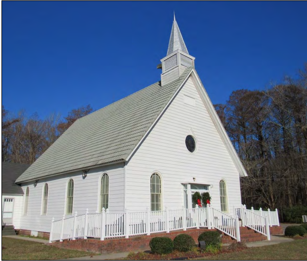
Photo 69: McBride United Methodist Church, South Oblique.
