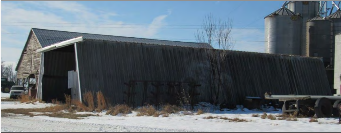
Photo 33: Circa-1980 Machine Shed, Northeast Oblique.
