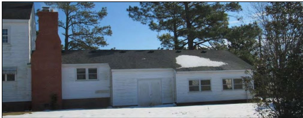
Photo 23: Circa-1985 Addition, West Elevation.
