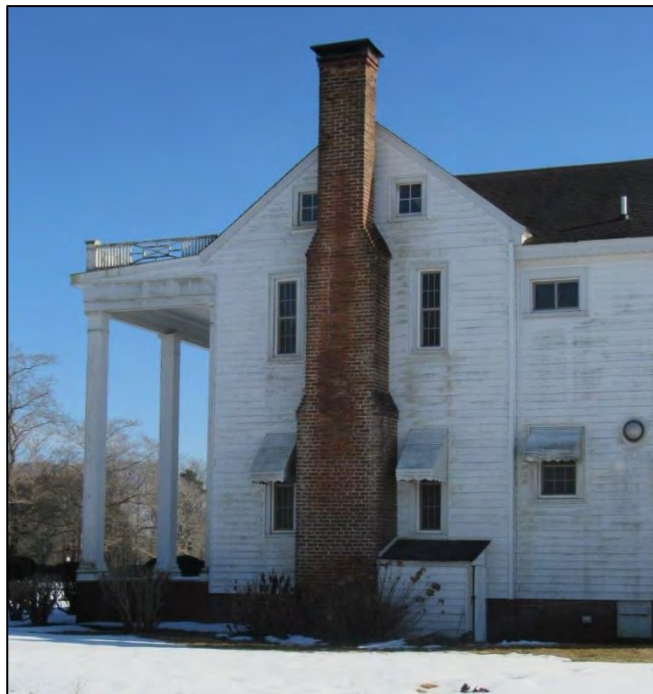
Photo 16: Double-Shouldered Chimney on the West Elevation.
