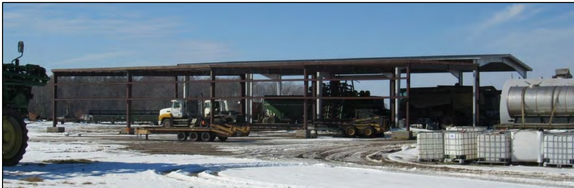
Photo 30: 2017 Equipment Shed (Foreground) and Circa-2000 Equipment Shed (Rear).
