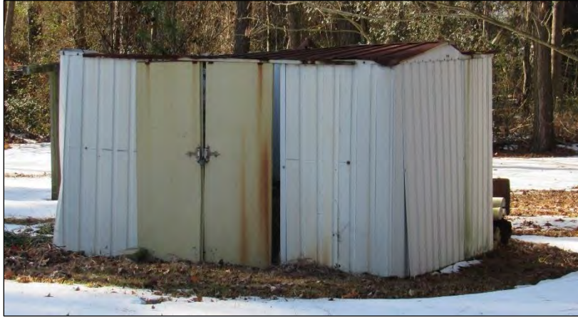
Photo 6: Shed, North Oblique.
