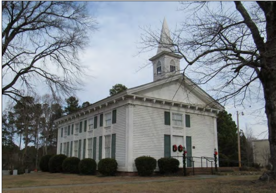
Photo 14: Forestville Baptist Church (WA0182), South Oblique.
