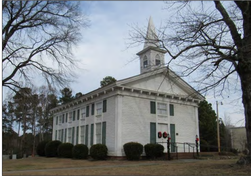
Photo 76: Forestville Baptist Church (WA0182), South Oblique.
