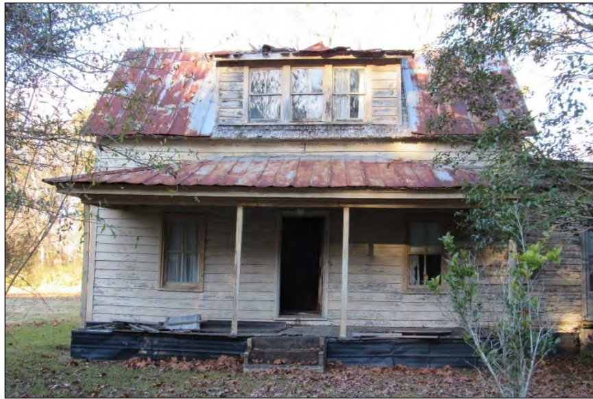
Photo 62: East Elevation of the Griffin House.
