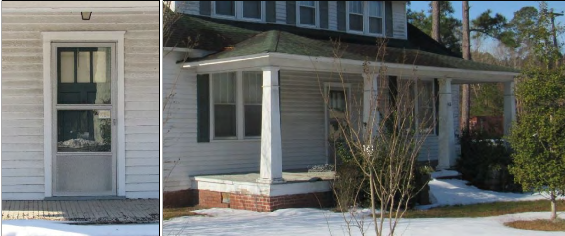
Photo 3: Detail of Primary Entrance (Left); Detail of Porch Along Façade (Right).
