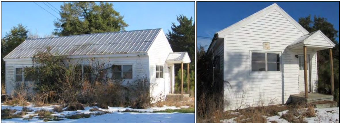
Photo 37: Circa-1950 Secondary Dwelling, Southwest Oblique (Left) and South Elevation (Right).
