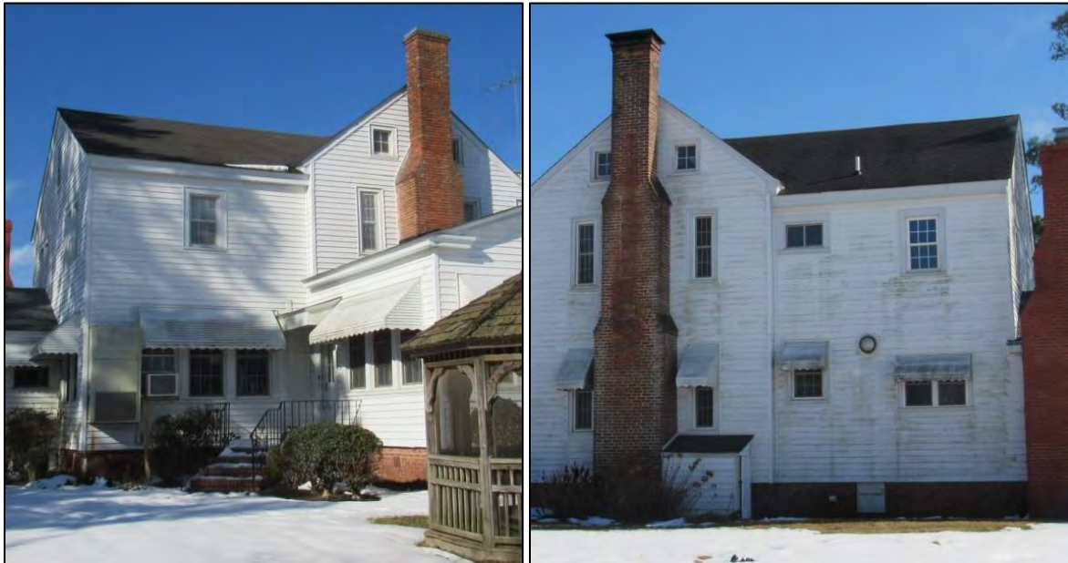
Photo 19: Rear Ell, East Elevation (Left) and West Elevation (Right).
