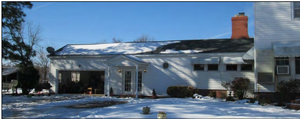
Photo 22: Circa-1985 Addition, East Elevation.
