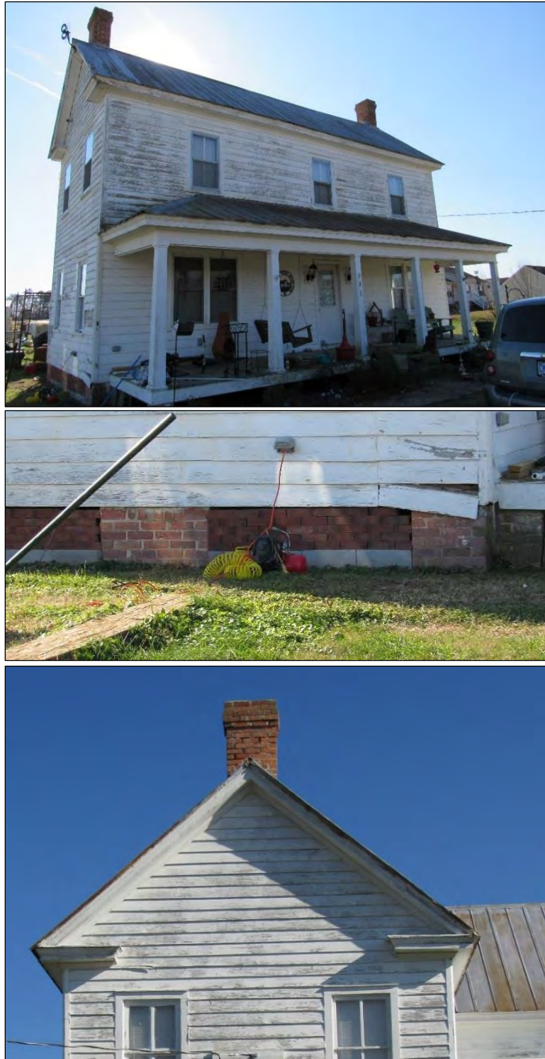
Photo 54: Northwest Elevation of the Pritchard House, Facing Southwest (Top); Detail of Foundation of Pritchard House, Northeast Elevation of Pritchard House (Middle); Detail of Gabled Returns and Chimney Flue, Southwest Elevation of Pritchard House (Bottom).
