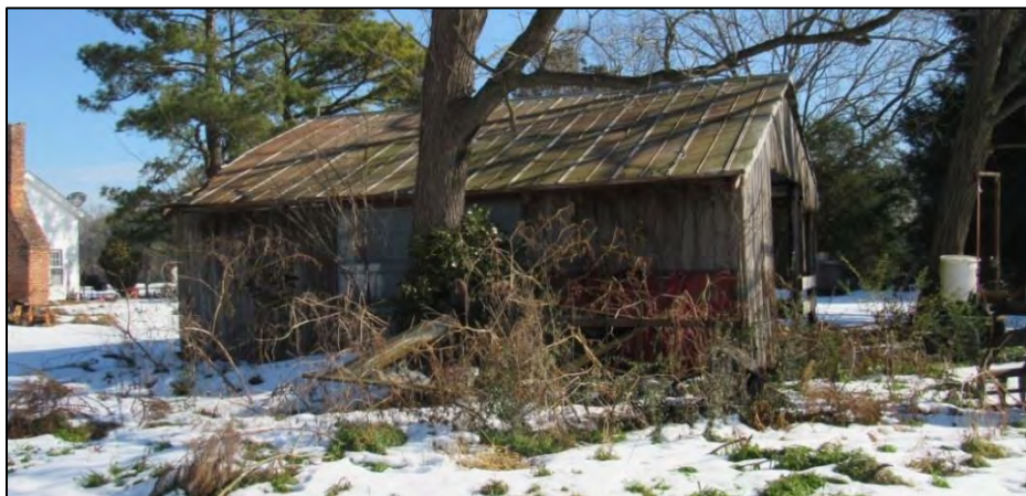
Photo 25: Circa-1950 Machine Shed, Southwest Oblique.
